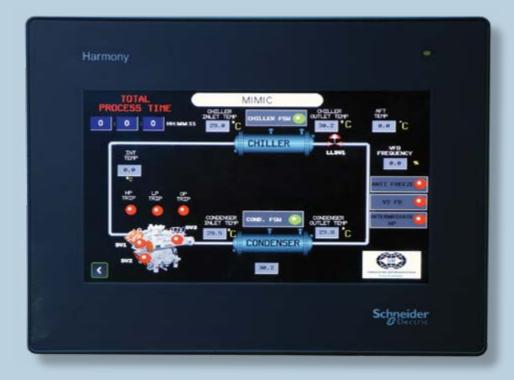
It can be challenging to monitor and control critical parameters in manual plants, such as suction superheat measurement, pressure controlling and level controls. We employ several components such as, electronic expansion valves, PLC, liquid level transmitters, motorized valves, level switches etc., that optimize your plant and make it the perfect solution for every process and all your requirements.
